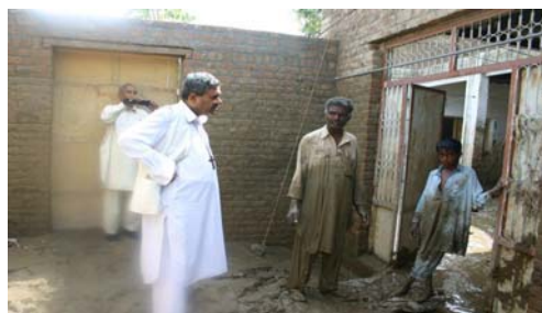
Bishop Humphrey inspecting a damaged house in Charsadda
