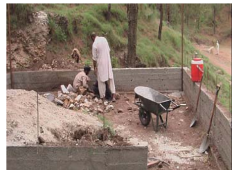
Local people of Pateka are busy in Construction Work
